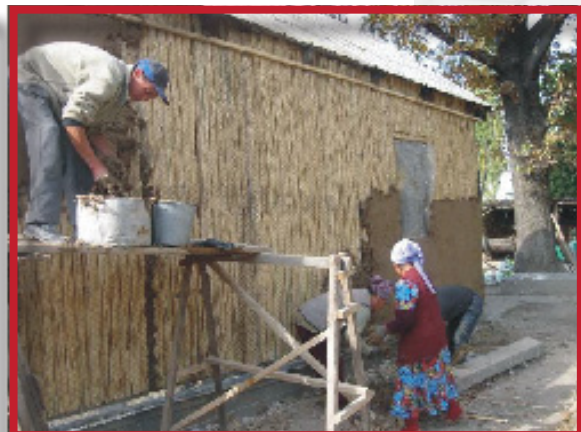
Plastering mat wall that made from reeds
