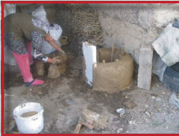
Construction of the second hearth
