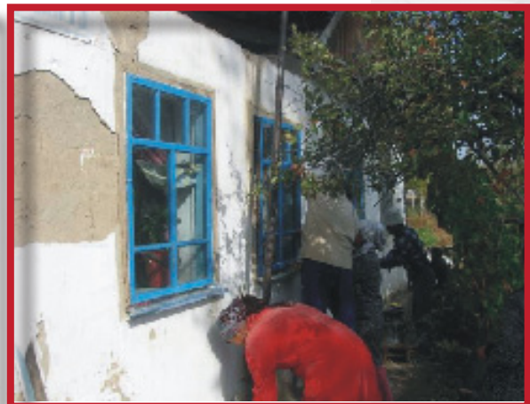
Air-tight installation of frames in window case
