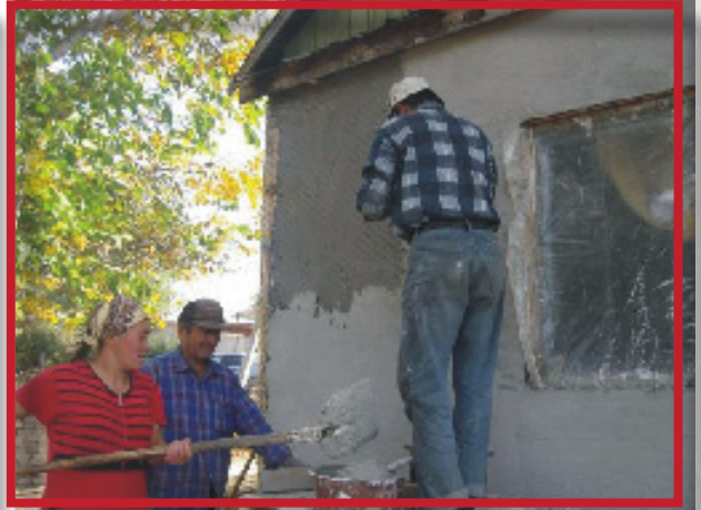
Placement of the heat-insulating material (foam plastic) in wooden frame made from strips Application of second layer of plaster out of lime-sand grout
