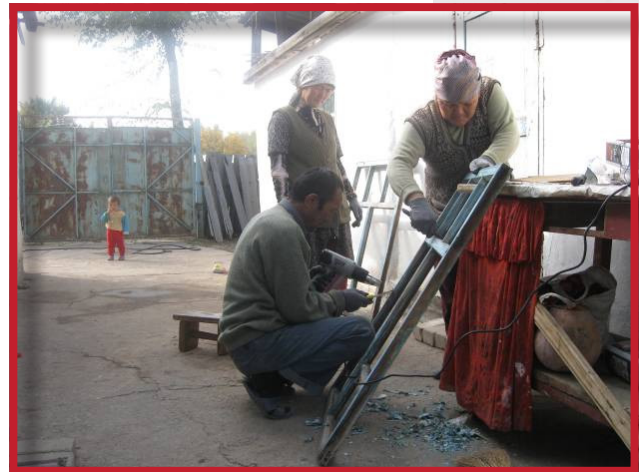
Preparation of old window frame
