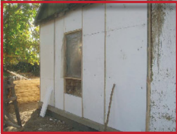
Placement of the heat-insulating material (foam plastic) in wooden frame made from strips Application of second layer of plaster out of lime-sand grout
