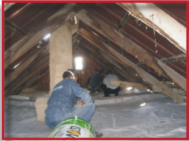
Laying vapor sealing and heat insulation material
