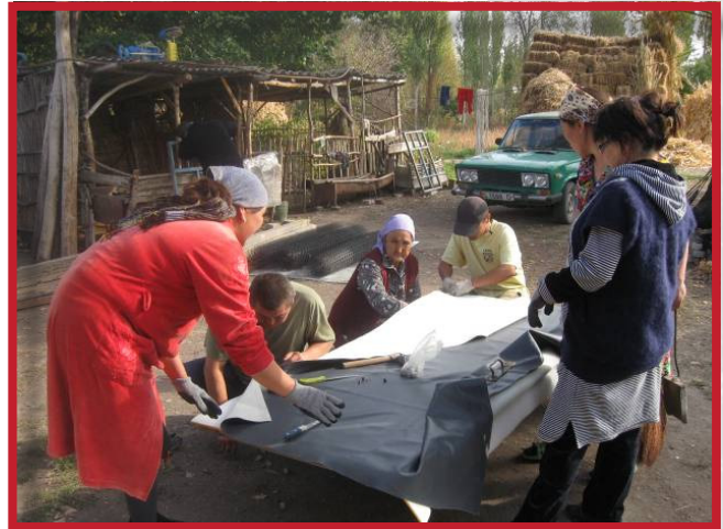
Heat –insulation of the external door
