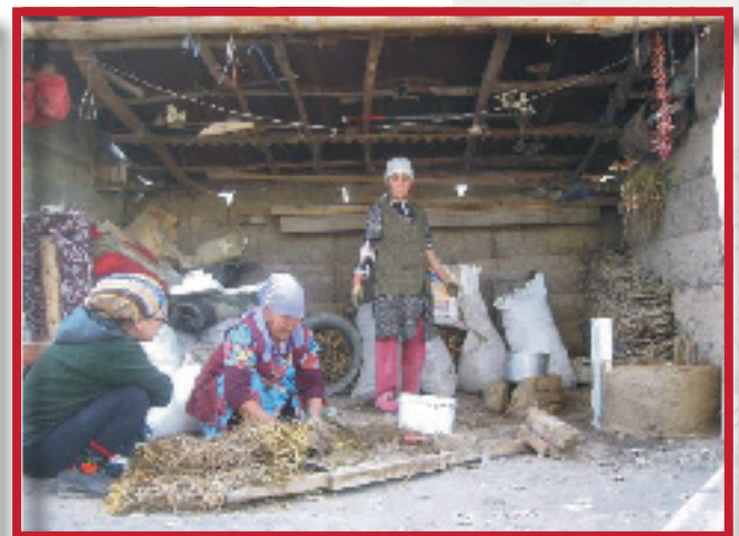
Clay and straw preparation to make a hearth
