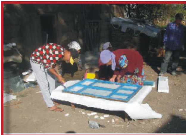
Air-tight glazing of a window frame
